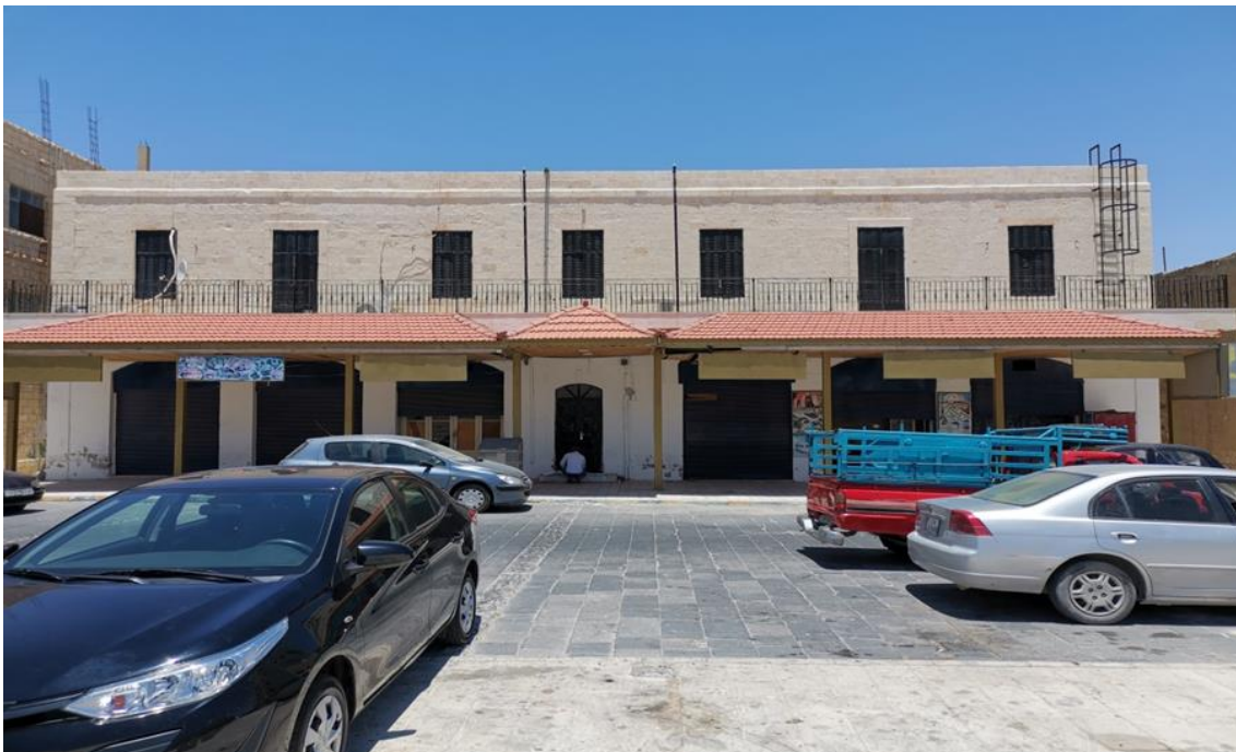
Picture 1: Front Elevation\ Southern Elevation of the mentioned building, June 2020
